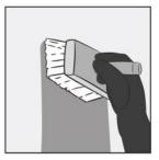
Apply the first coat of TAL SUREPROOF SHOWER to the clean, dry, primed surface with a block brush and allow to dry (approximately 1-2 hours).
